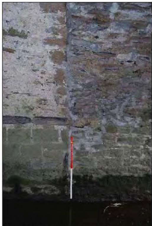
**Plate 36:** Transition-point between mid-section (Phase 1) and downstream section (Phase 2), north side of **Arch no. 4** (1m scale).
