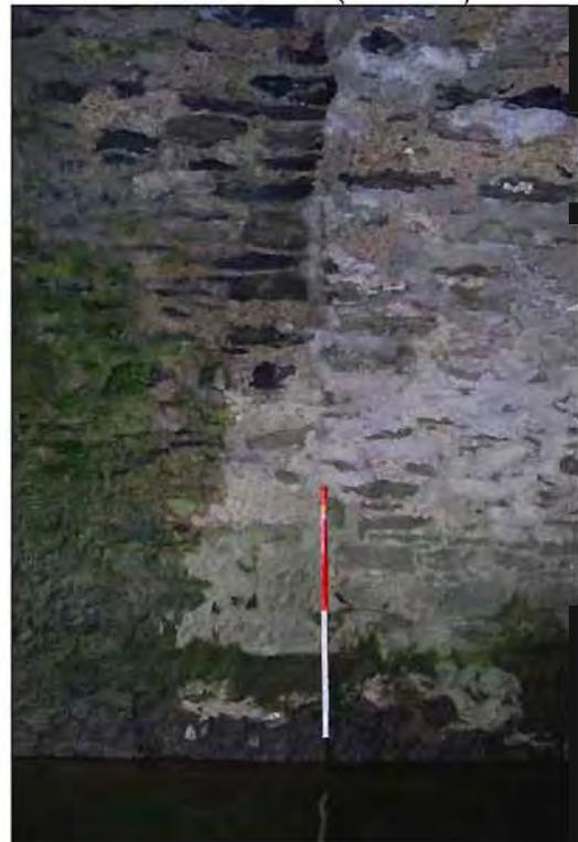
**Plate 26:** Transition-point between mid-section (Phase 1) and upstream section (Phase 2), north side of **Arch no. 4** (1m scale).
