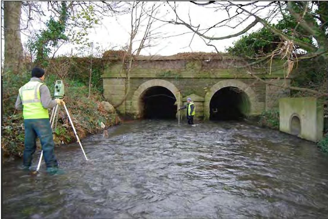
**Plate 9:** Working-shot of Total Station survey undertaken along upstream side of Balheary Bridge (Feature 3), Ward River.
