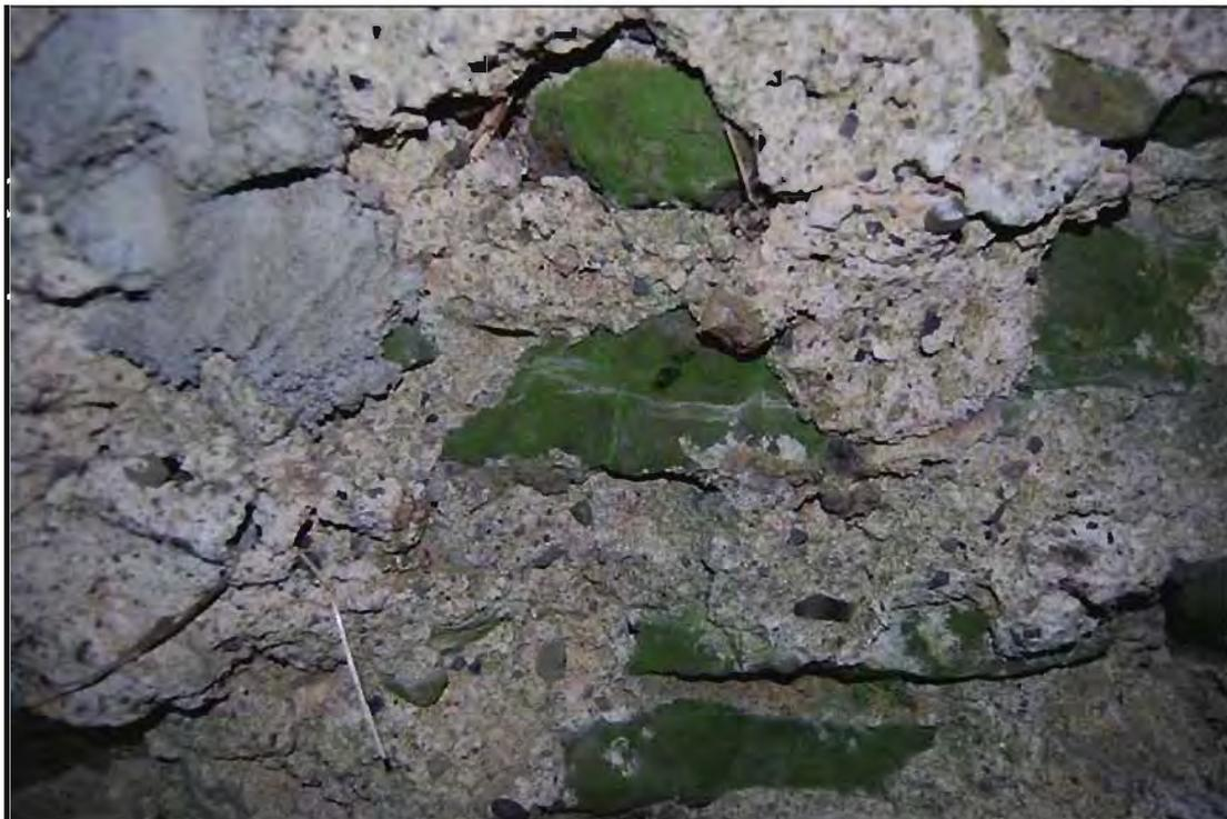
**Plate 76:** Detail shot of mortar located across intrados of middle section (Phase 1) of Arch nos. 1 and 2 from Balheary Bridge (Feature 3).
