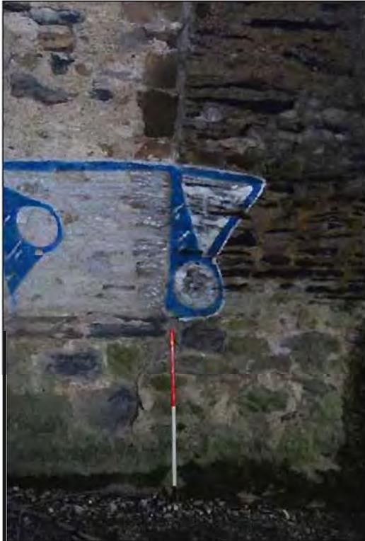
**Plate 23:** Transition-point between mid-section (Phase 1) and upstream section (Phase 2), south side of **Arch no. 3** (1m scale).
