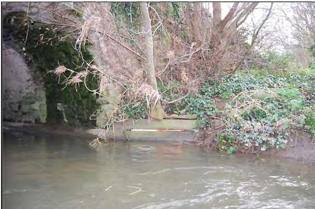
**Plate 68:** Southeast-facing view of concrete encased bridge footings located along the base of **Arch no. 1**, upstream side of Lissenhall Bridge, Feature 1 (1m scale).
