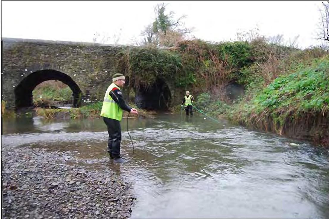
**Plate 5:** Working-shot of diver undertaking riverbed survey along downstream side of Lissenhall Bridge, northern flow-channel of Broadmeadow River. Note: diver tethered to counteract against river-flow.
