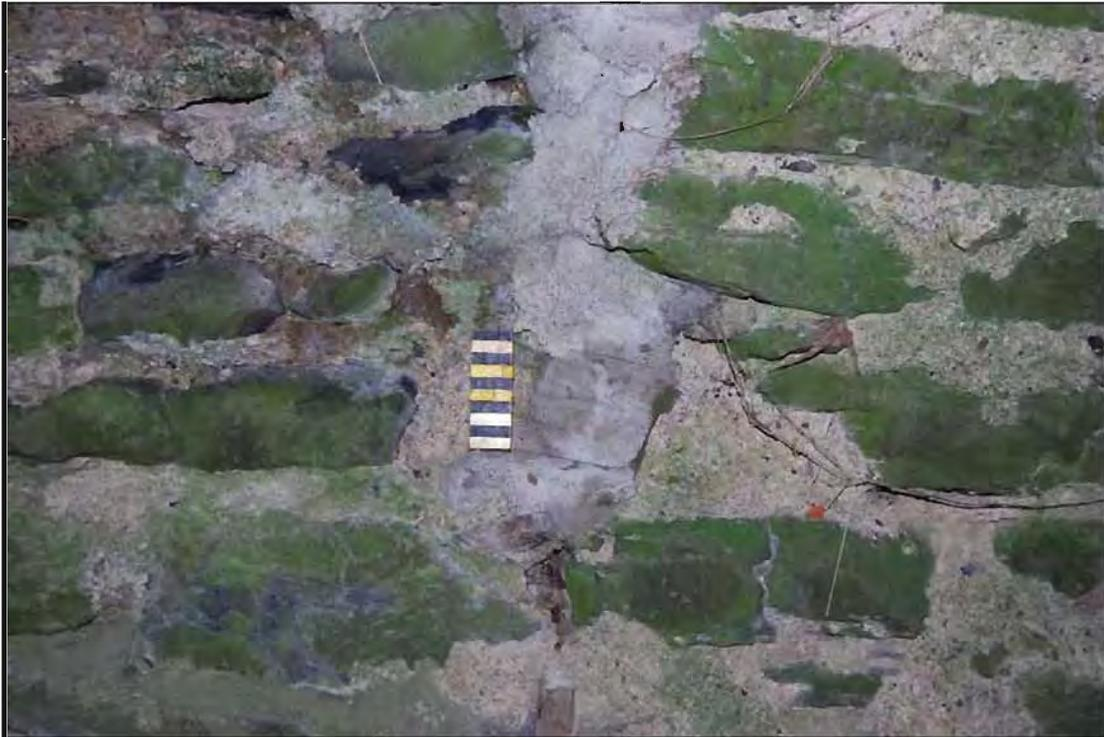
**Plate 53:** Detail shot of intrados transition-point between the upstream section (Phase 2) and the middle section (Phase 1) from **Arch no. 1**, Lissenhall Bridge, Feature 1 (10cm scale).
