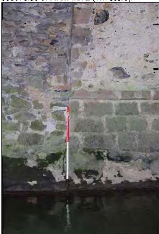
**Plate 33:** Transition-point between mid-section (Phase 1) and downstream section (Phase 2), south side of **Arch no. 3** (1m scale).
