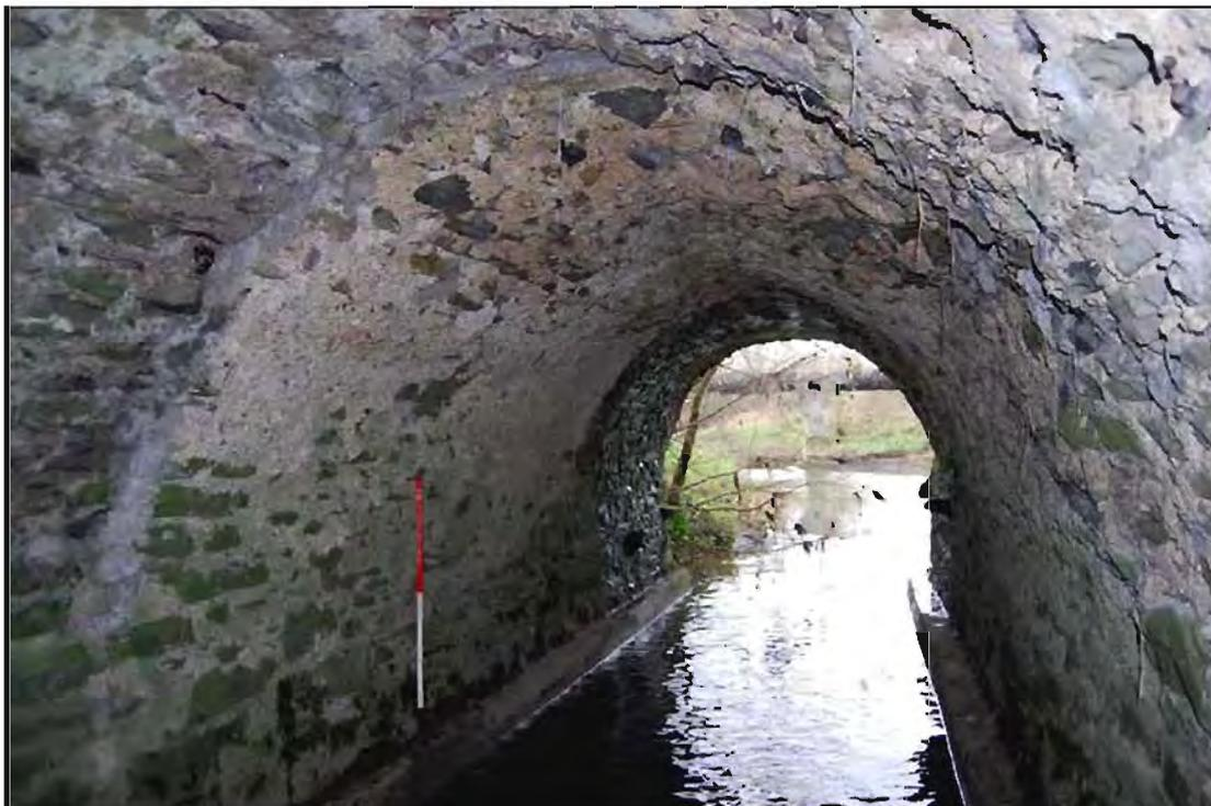
**Plate 52:** West-facing view across arch-ceiling (intrados) of Arch no. 1, Lissenhall Bridge (Feature 1). Note: differing composition of intrados and concrete underpinning of bridge footings (1m scale).
