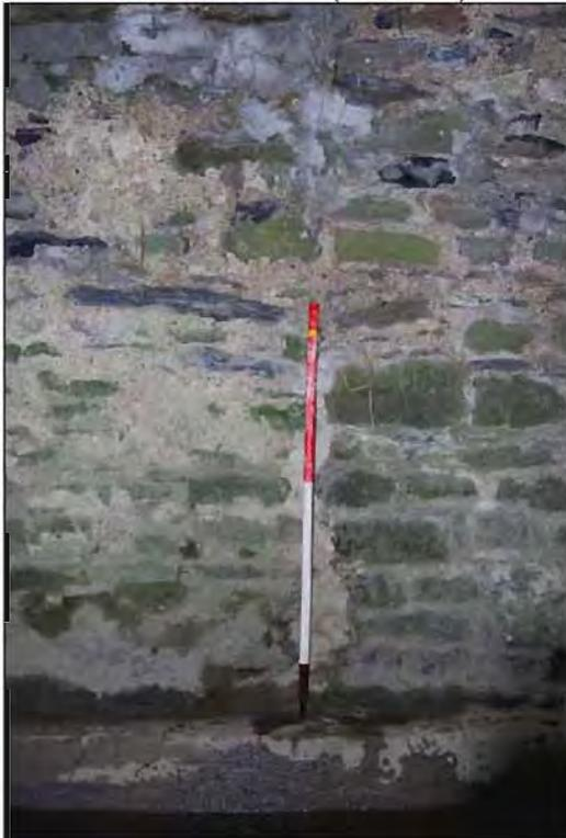
**Plate 29:** Transition-point between mid-section (Phase 1) and downstream section (Phase 2), south side of **Arch no. 1** (1m scale).
