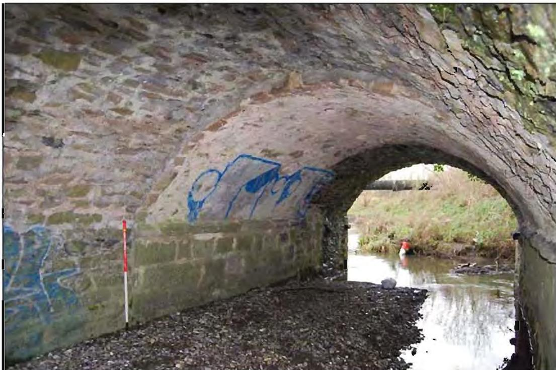
**Plate 58:** Southwest-facing view across arch-ceiling (intrados) of Arch no. 3, Lissenhall Bridge (Feature 1). Note: differing composition of intrados and protruding arch-stones from downstream side of mid-section (1m scale).
