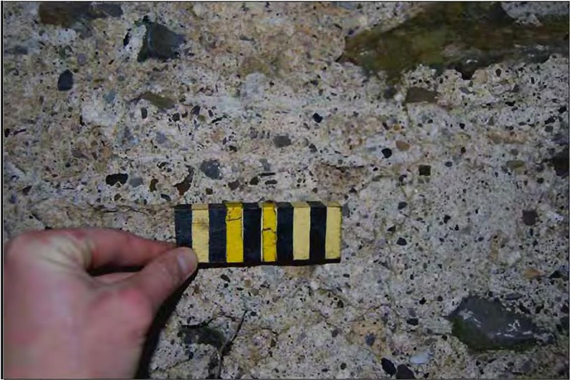
**Plate 41:** Detail shot of coarse mortar covering the intrados of the mid-section of Lissenhall Bridge. (10cm scale).
