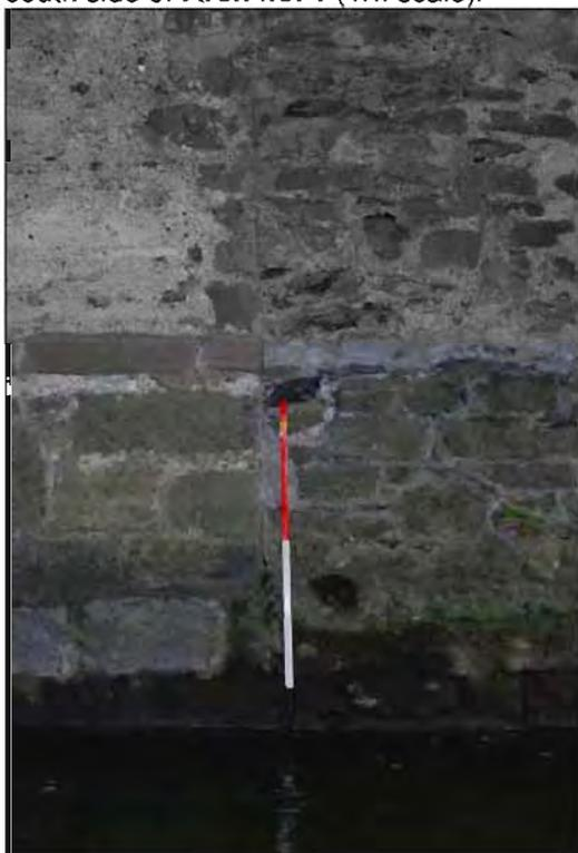
**Plate 21:** Transition-point between mid-section (Phase 1) and upstream section (Phase 2), south side of **Arch no. 2** (1m scale).
