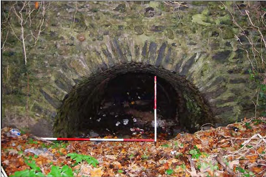
**Plate 69:** East-facing view of the single-arched culvert comprising Feature 2, located approximately mid-point between Lissenhall Bridge, Feature 1, and Balheary Bridge, Feature 3 (1m vertical and 2m horizontal scale).
