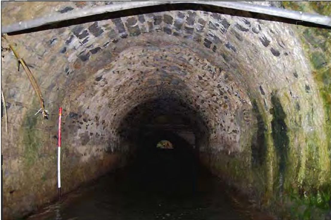
**Plate 77:** East-facing view through **Arch no. 1** showing transition between the upstream (Phase 3) and middle section (Phase 1) at Balheary Bridge, Feature 3 (1m scale).
