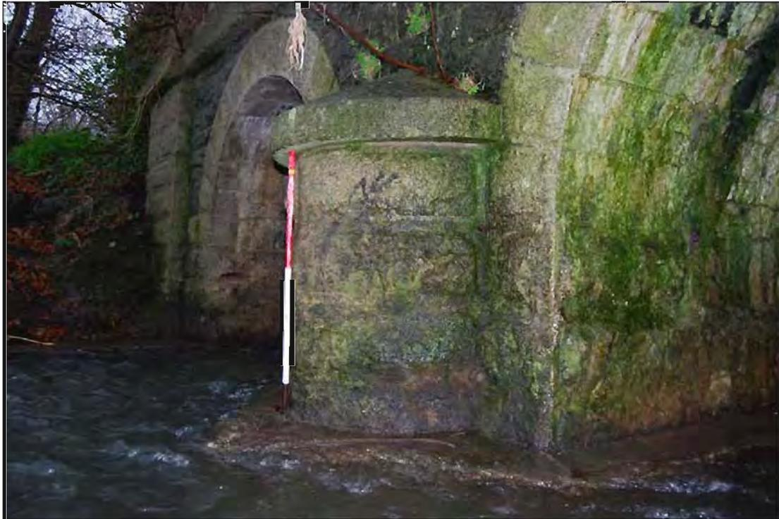
**Plate 81:** North-facing view of semi-circular cutwater located between Arch nos. 1 and 2 on upstream side of Balheary Bridge, Feature 3 (1m scale). Note: concrete underpinning of bridge structure.
