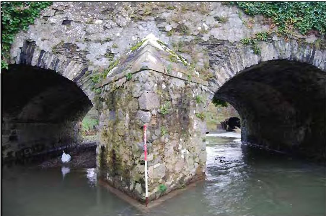
**Plate 48:** East-facing view of Cutwater No. 2, located between Arch nos. 2 and 3, Lissehanll Bridge, Feature 1 (1m scale).
