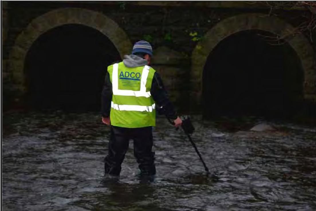
**Plate 7:** Working-shot of metal-detector survey undertaken across upstream side of Balheary Bridge, Ward River.
