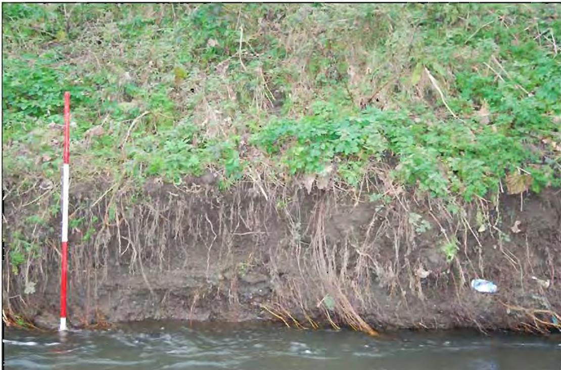
**Plate 12:** North-facing view of bankside erosion taking place along the base of the northern bank structure, downstream side of Lissenhall Bridge, Broadmeadow River (2m scale).
