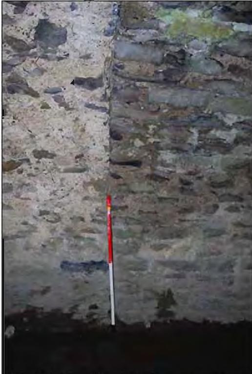
**Plate 27:** Transition-point between mid-section (Phase 1) and upstream section (Phase 2), south side of **Arch no. 5** (1m scale).
