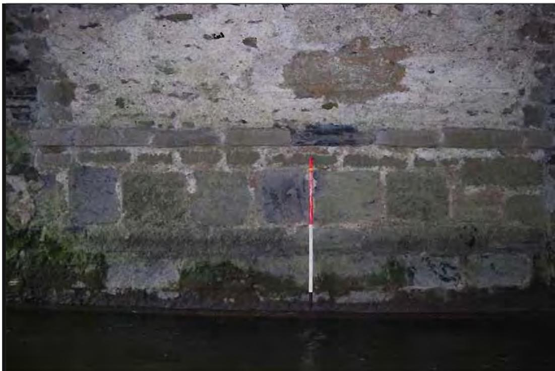
**Plate 43:** North-facing view of arch wall from the re-built mid-section, north side of Arch no. 2, Lissenhall Bridge, Feature 1 (1m scale).
