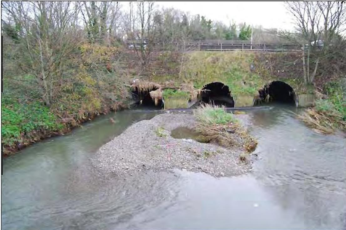
**Plate 1:** East-facing view of downstream side of Lissenhall Bridge showing pebble island and three-arched culvert that accommodates the N1 Link-Road (1m horizontal and 2m vertical scale).
