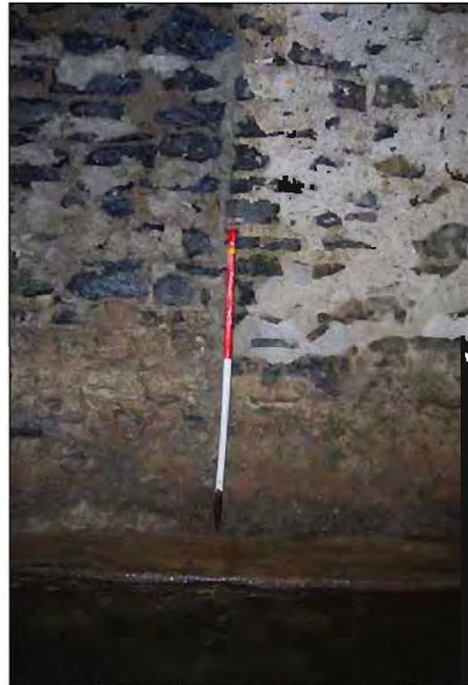
**Plate 75:** Transition-point between mid-section (Phase 1) and downstream section (Phase 2), north side of Arch no. 2 (1m scale).
