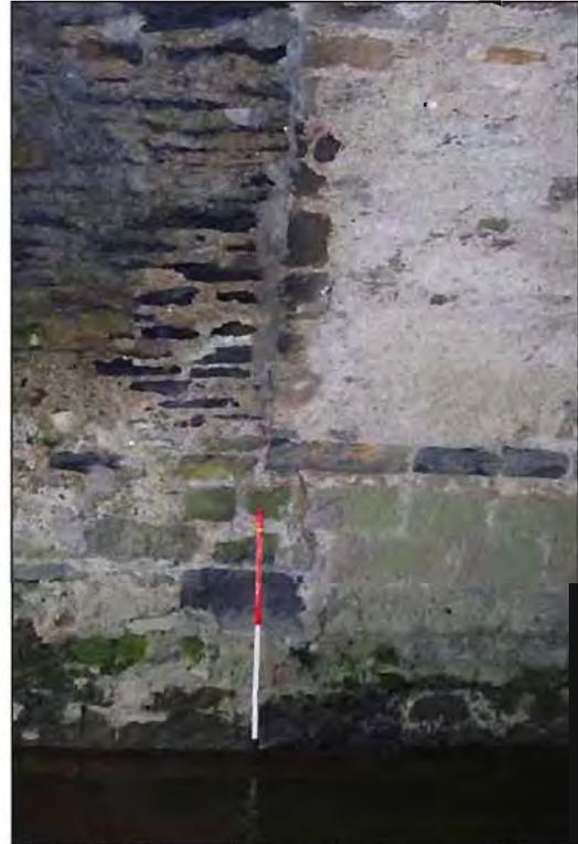
**Plate 24:** Transition-point between mid-section (Phase 1) and upstream section (Phase 2), north side of **Arch no. 3** (1m scale).
