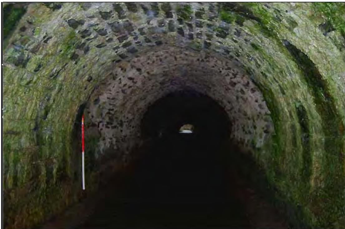
**Plate 78:** East-facing view through **Arch no. 2** showing transition between the upstream (Phase 3) and middle section (Phase 1) at Balheary Bridge, Feature 3 (1m scale).
