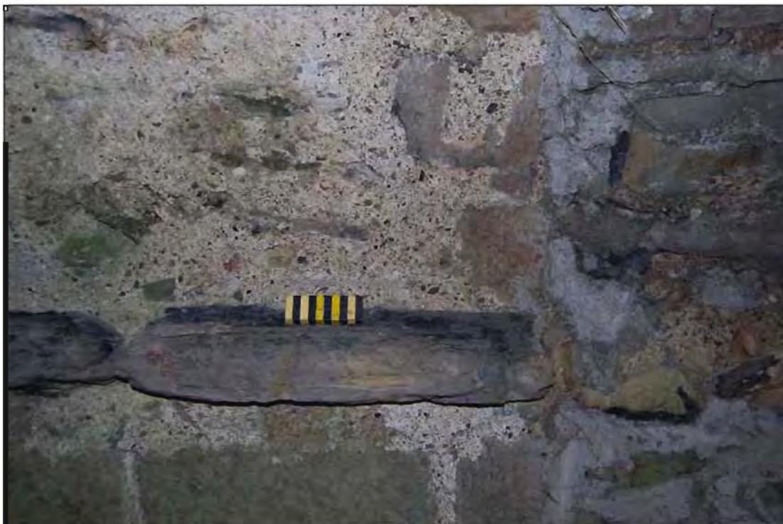
**Plate 45:** North-facing view across lintel forming at top of arch-wall on north side of the mid-section of **Arch no. 2**, Lissenhall Bridge, Feature 1 (10cm scale).
