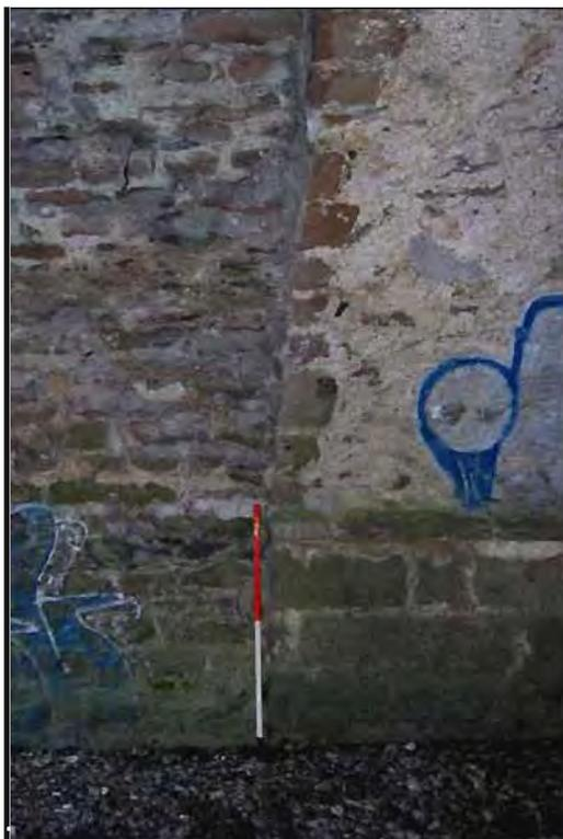
**Plate 35:** Transition-point between mid-section (Phase 1) and downstream section (Phase 2), south side of **Arch no. 4** (1m scale).
