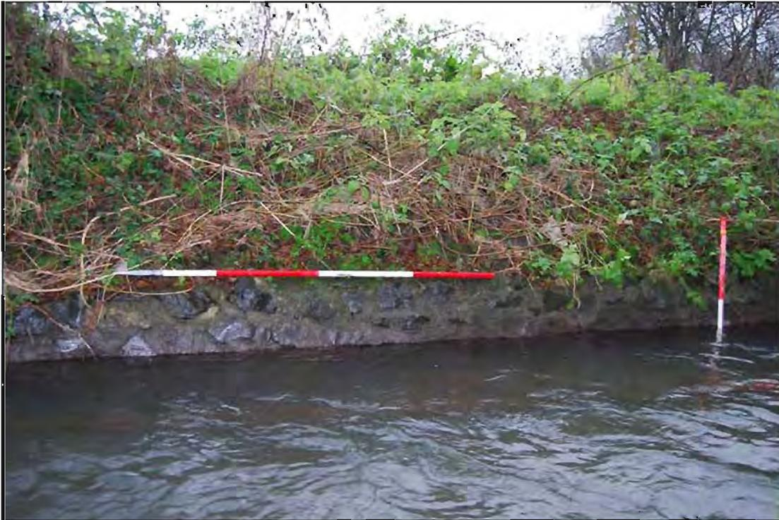
**Plate 85:** North-facing detail shot of revetment wall (Feature 5, Section 1) located along north side of the river (1m vertical and 2m horizontal scale).
