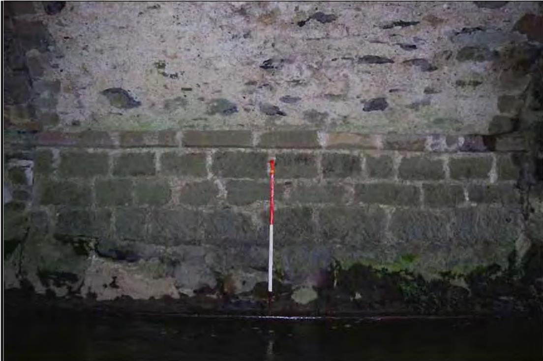
**Plate 42:** South-facing view of arch wall from the re-built mid-section, south side of Arch no. 2, Lissenhall Bridge, Feature 1 (1m scale).
