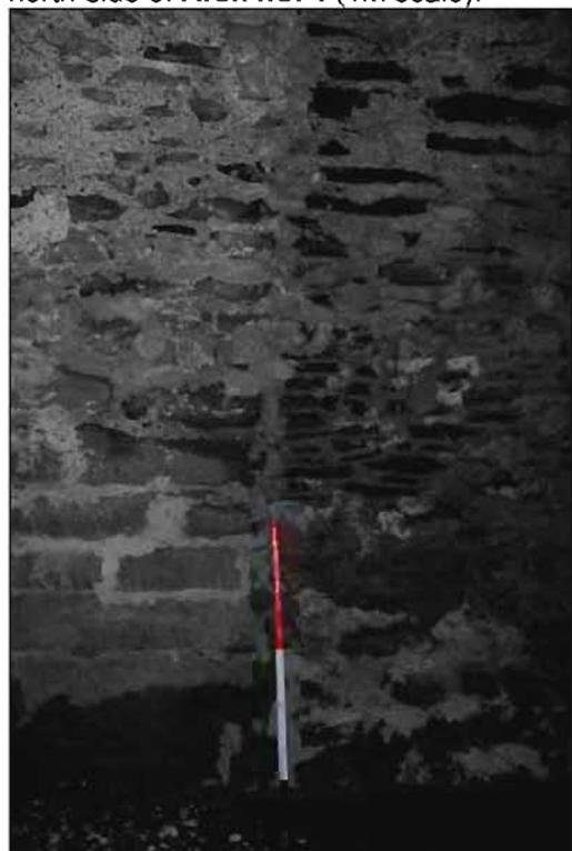
**Plate 38:** Transition-point between mid-section (Phase 1) and downstream section (Phase 2), north side of **Arch no. 5** (1m scale).
