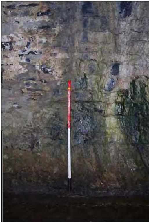
**Plate 72:** Transition-point between mid-section (Phase 1) and upstream section (Phase 3), north side of Arch no. 1 (1m scale).
